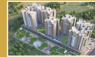
ATHARVA NAGARI - VII Near Besa Square, Nagpur (Work in Progress)
